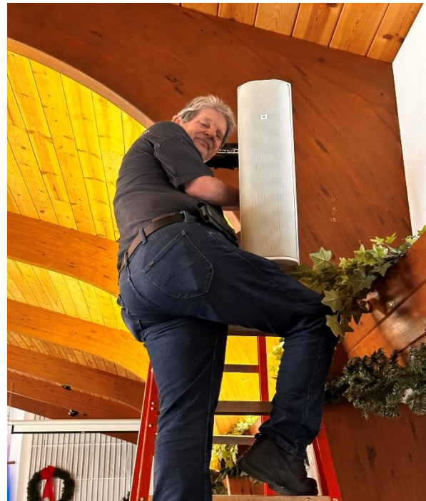
John installing of o four new Bose speakers
